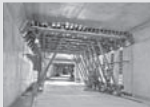
Tunnel Formwork
