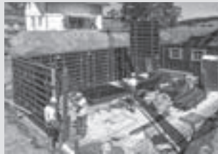
Wall Formwork
