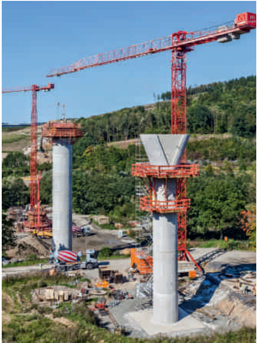
The SCS provided the optimum solution for the heads of these reinforced concrete piers for the composite bridge.
