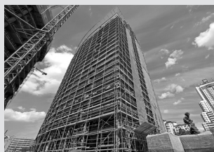
Facade working scaffold
