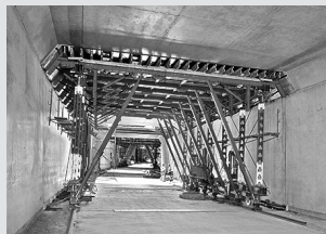
Tunnel formwork
