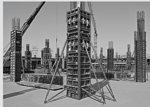
Column formwork
