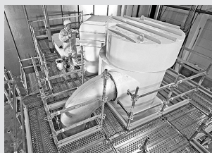
Working scaffolds industry
