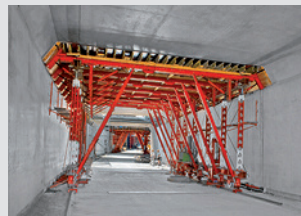
Tunnel Formwork
