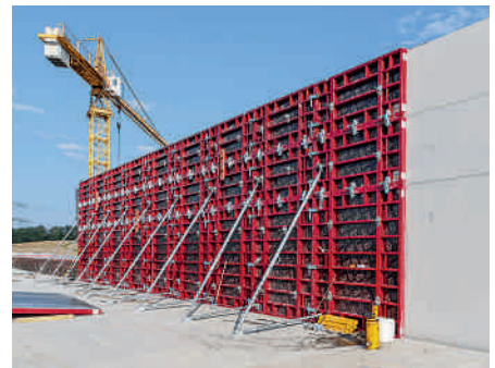
... and installation at the required position.
