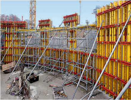
Use with VARIO GT 24 Girder Wall Formwork The Arctic Ring, Copenhagen Zoo, Denmark.
