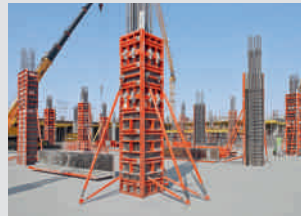
Column Formwork
