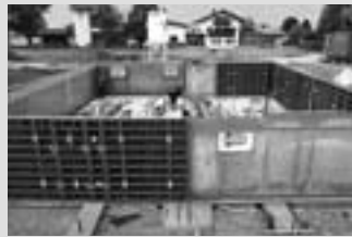
Wall Formwork
