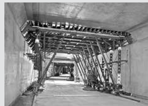
Tunnel Formwork
