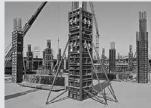
Column Formwork
