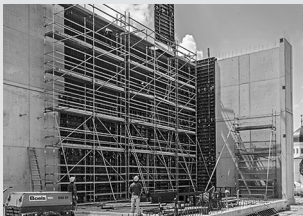
Working scaffolds construction
