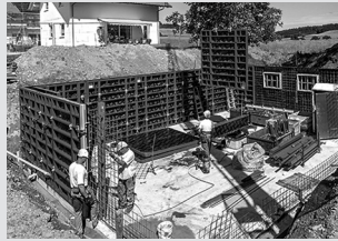
Wall formwork
