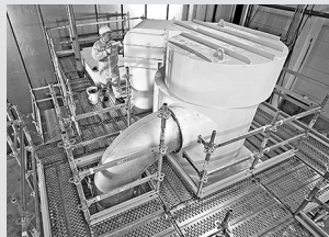
Working scaffolds industry
