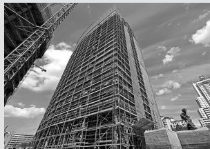
Working scaffolds facade
