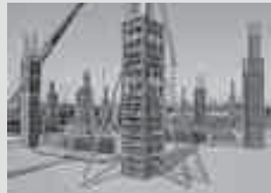
Column Formwork
