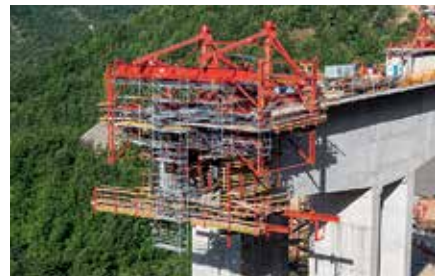
Safe access means Modular working platforms and access to all working areas due to the compatibility with PERI UP.
