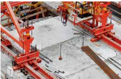
Lower workload Only 2 anchors per A-frame required.
