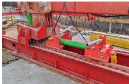
No unintentional movement The equipment is always mechanically secured when being moved forward to the next cycle.
