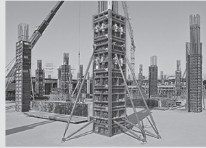
Column Formwork
