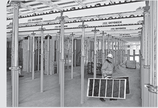
Slab Formwork
