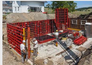
Wall Formwork
