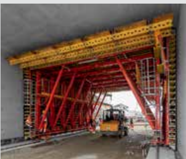
Cut-and-cover, semi-monolithic construction method
