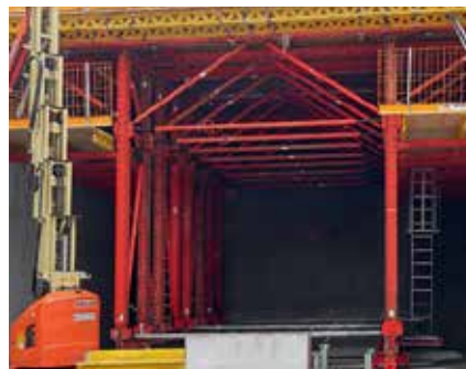
In accordance with the occurring loads, it is possible to realise supporting structures with diagonal struts or trusses with the Vertical Post.
