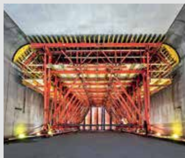
Cut-and-cover, separate casting method
