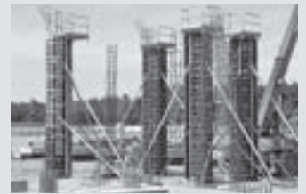
Column Formwork
