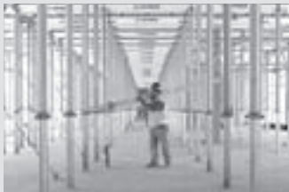
Slab Formwork
