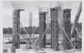
Column Formwork
