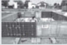
Wall Formwork
