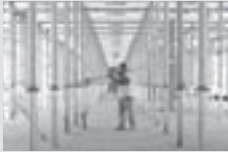
Slab Formwork
