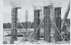
Column Formwork
