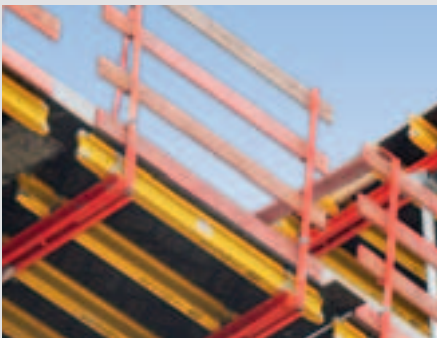
By means of the Guardrail Holder SRU/SRZ and the Guardrail Post SGP, guardrails on the slab edge are mounted.
