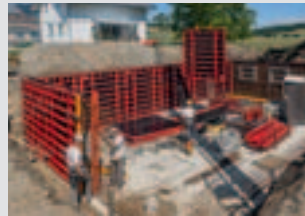
Wall Formwork
