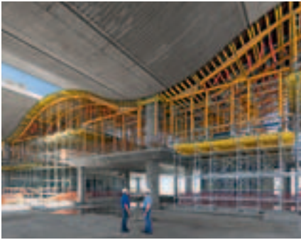
VARIOKIT and MULTIPROP system components formed the cost-effective basis for the form-shaping slab tables.
