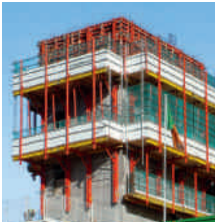
With the RCS Rail Climbing System, different wall formwork systems are used as well as the proven TRIO panel formwork.
