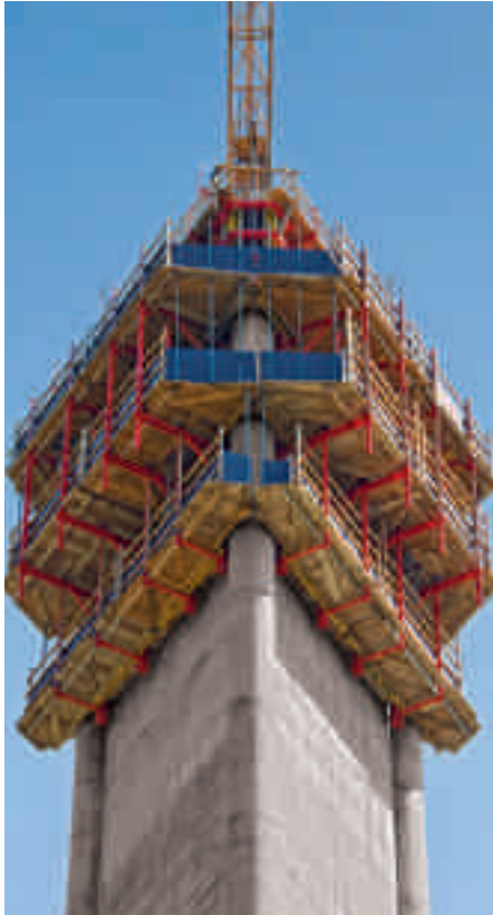
As an alternative to complete enclosure, scaffold tubes or handrail boards also provide safe lateral protection.
