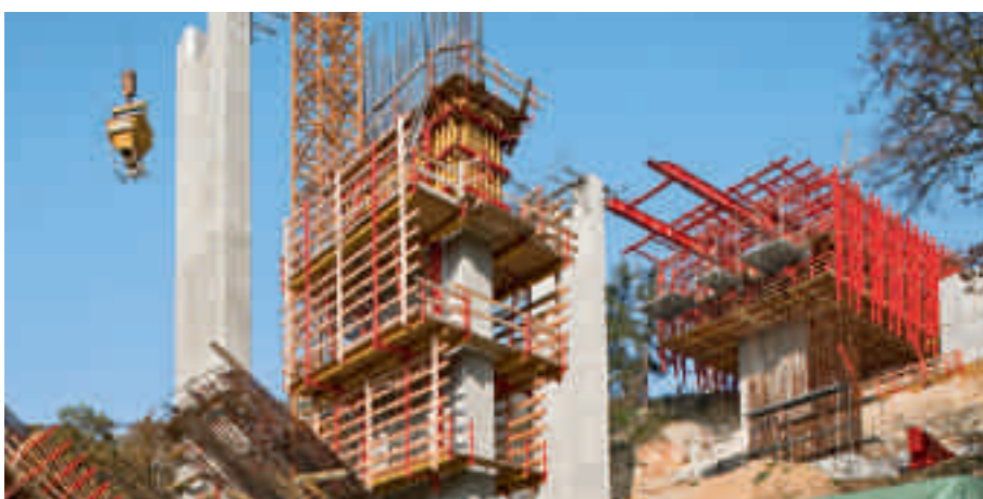
Another typical area of application for the RCS Rail Climbing System is bridge piers.
