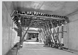
Tunnel Formwork
