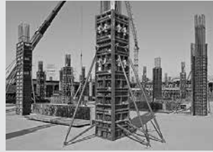
Column Formwork
