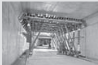
Tunnel Formwork
