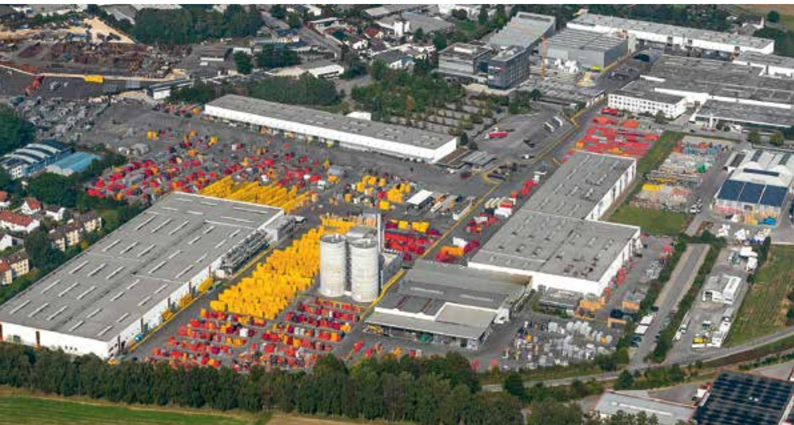
PERI in Weissenhorn: company headquarters, development and production.
